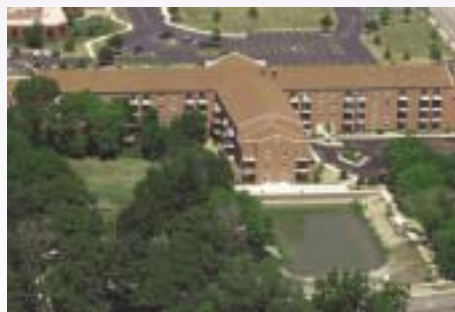
Library Lane: This senior housing in Grayslake, IL, is a 148-unit complex which was built utilizing tax credits. Class A rating.
