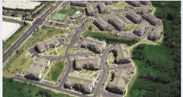
Osprey Lake Apartments: Located in Gurnee, IL, this two-phase, luxury, 483 unit development is located on 88 acres of lush forest and wetlands. A gated community with indoor and outdoor pools, clubhouse with exercise facility, tennis courts, wooded jogging path, and private 15-acre stocked lake. Class A+ rating.
